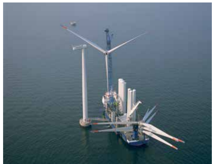
Marine wind turbine under construction off the coast of Denmark.
